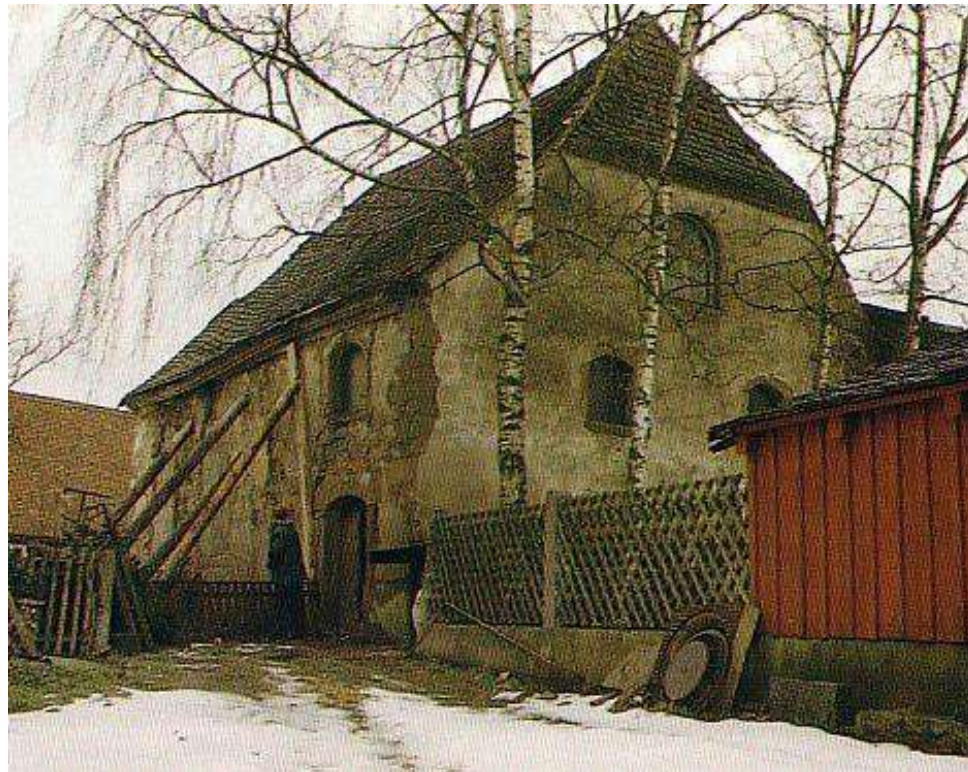
Michelbach Synagogue before restoration
