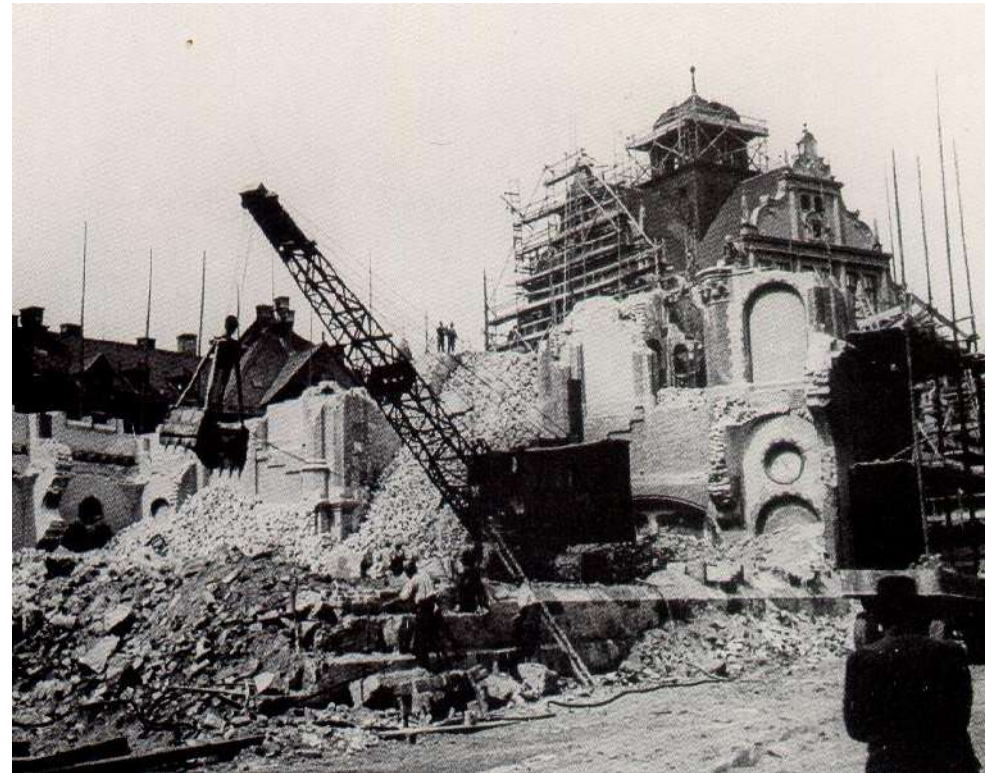
Main Synagogue Munich, Demolition summer 1938
