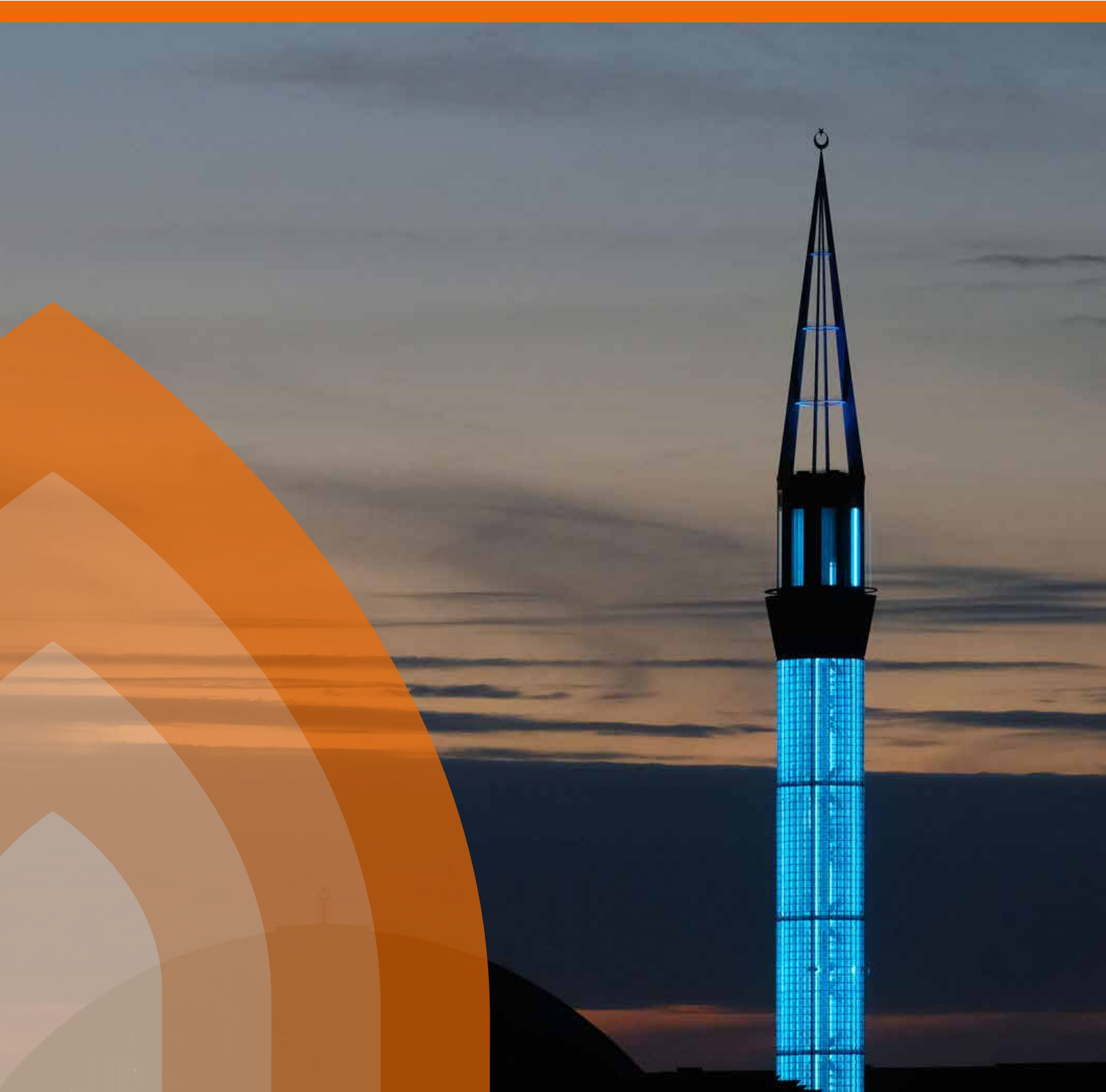
© image: Ter Brake A.B. - Mosque Utrecht - The Netherlands
