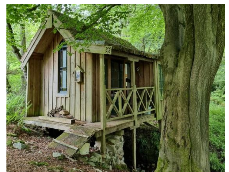
Fig. 2, 3, 4 Images of a Monastic Settlement in Shropshire
