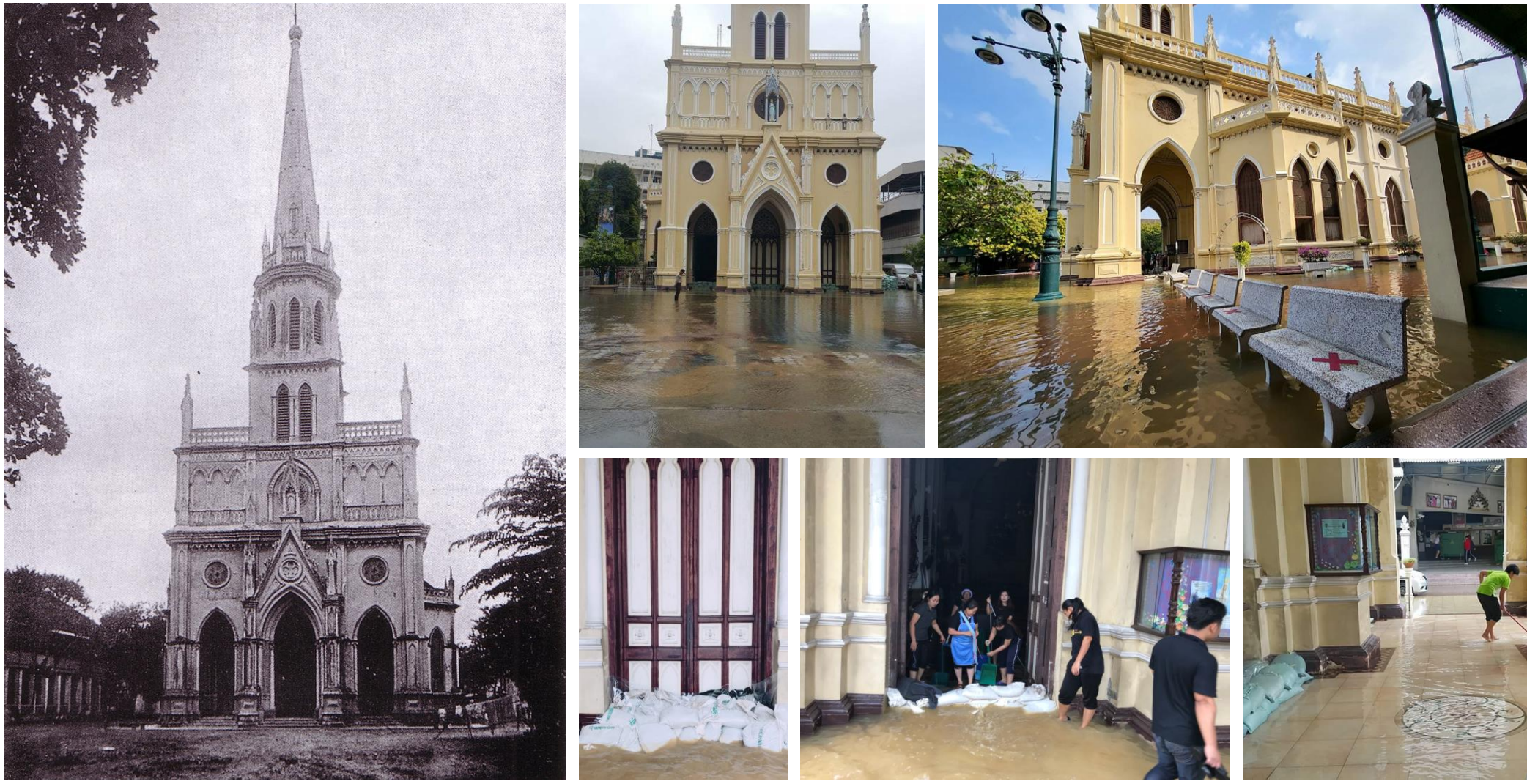
Fig.5 The Holy Rosary Church with the staircase at the porch, c.1908. (Wright, A. 1908) Fig.6-10 Porch of the Holy Rosary Church during flooding season with sandbags, temporary path and volunteers, 2022. Currently, the interior floor level of the Holy Rosary Church is the lowest point on the property, which was the result of consistently filling up the surrounding landscape to avoid flood. However, this increases the risk of flooding as there needs to be a retention area for water.
