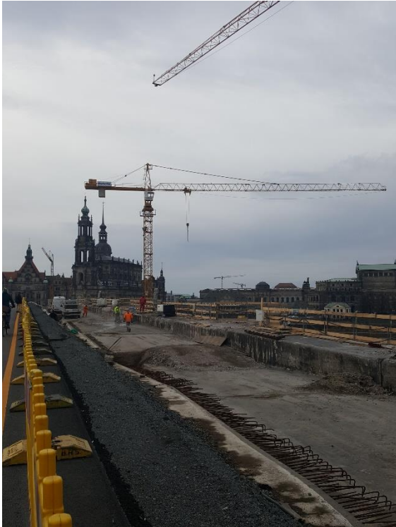
Figure 1. Constructing a new bridge towards heritage conservation.
