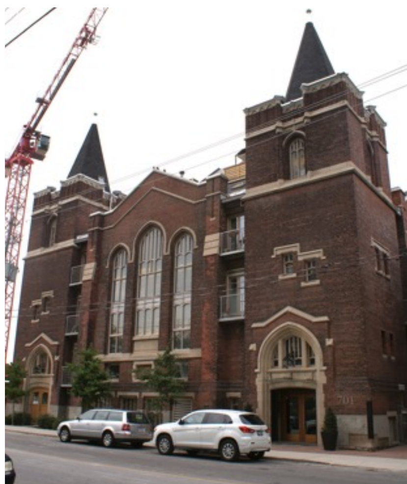
The Church Lofts 701 Dovercourt Road
