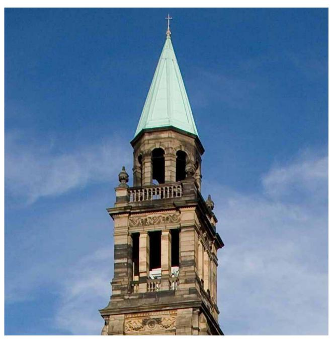
Tower of St George's West Church, Shandwick Place, Edinburgh. Telecommunications transmitters disguised as stonework – note the fattened profiles of the central columns at the first open stage of the tower.
