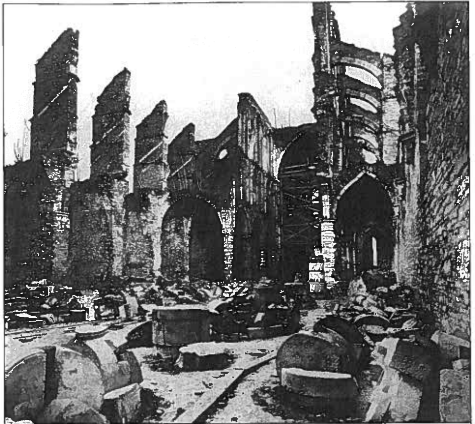
Ill. 5: The first stage of restoration consisted in cleaning the site and sorting the stones, which could be reused for anastylosis. Nave of the church, December 1893.
